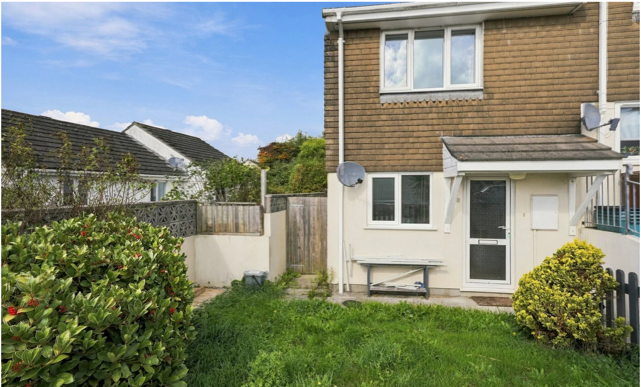
Vincent's Road, Kingsbridge Kingsbridge
