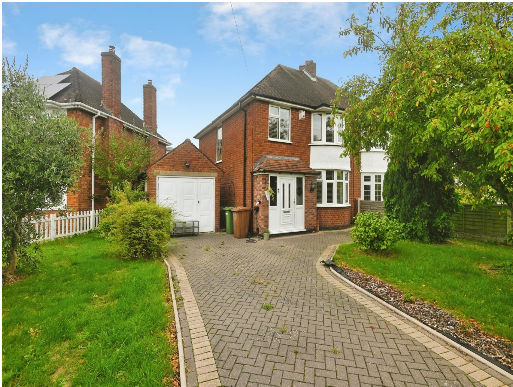
Marlborough Road, Castle Bromwich Birmingham B36 0EL
