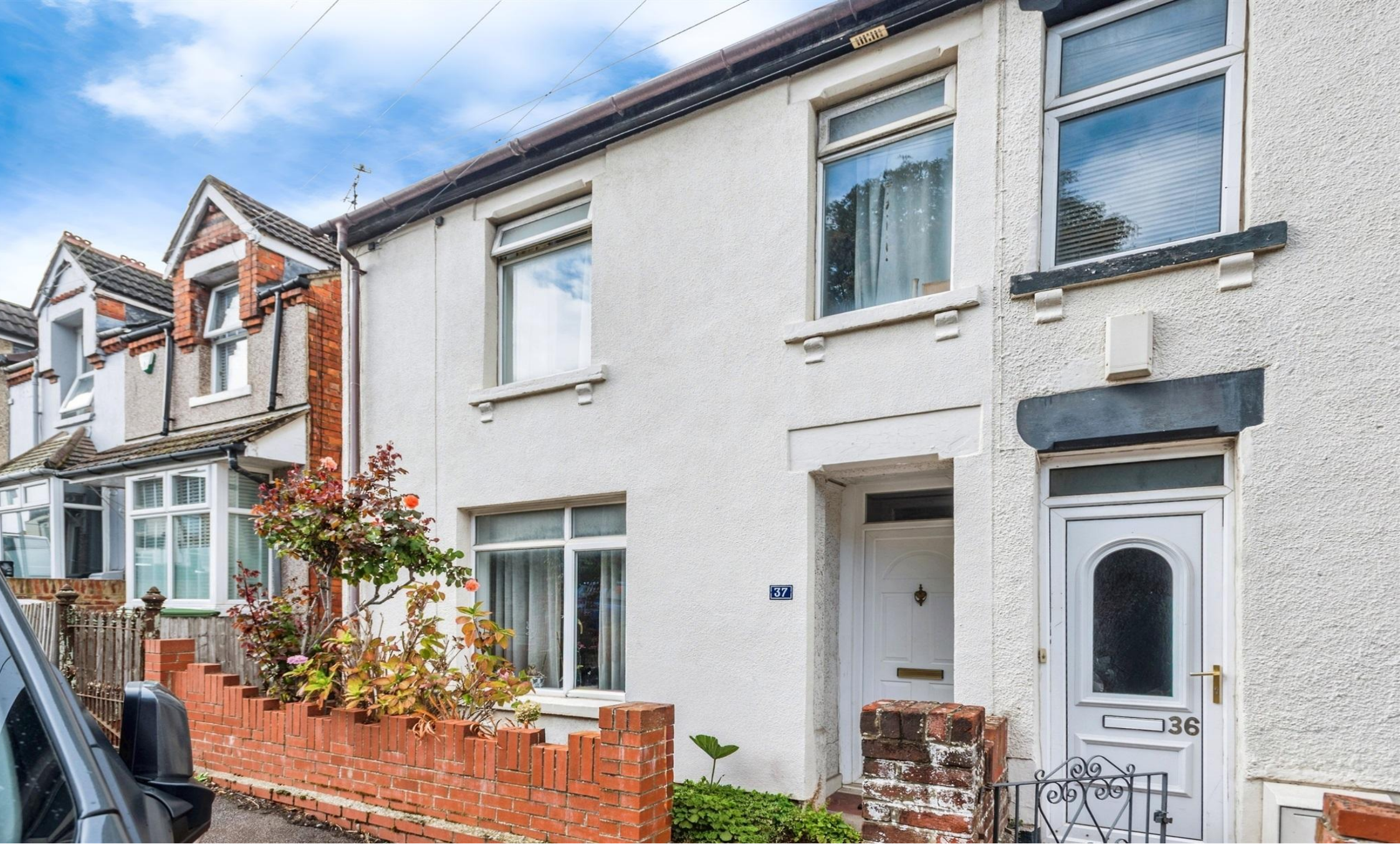
Radnor Street, Swindon, SN1 3PR
