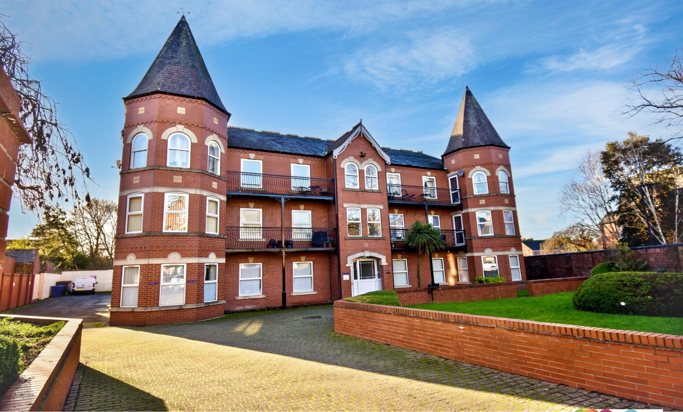
Auckland Grange Auckland Road, Doncaster
