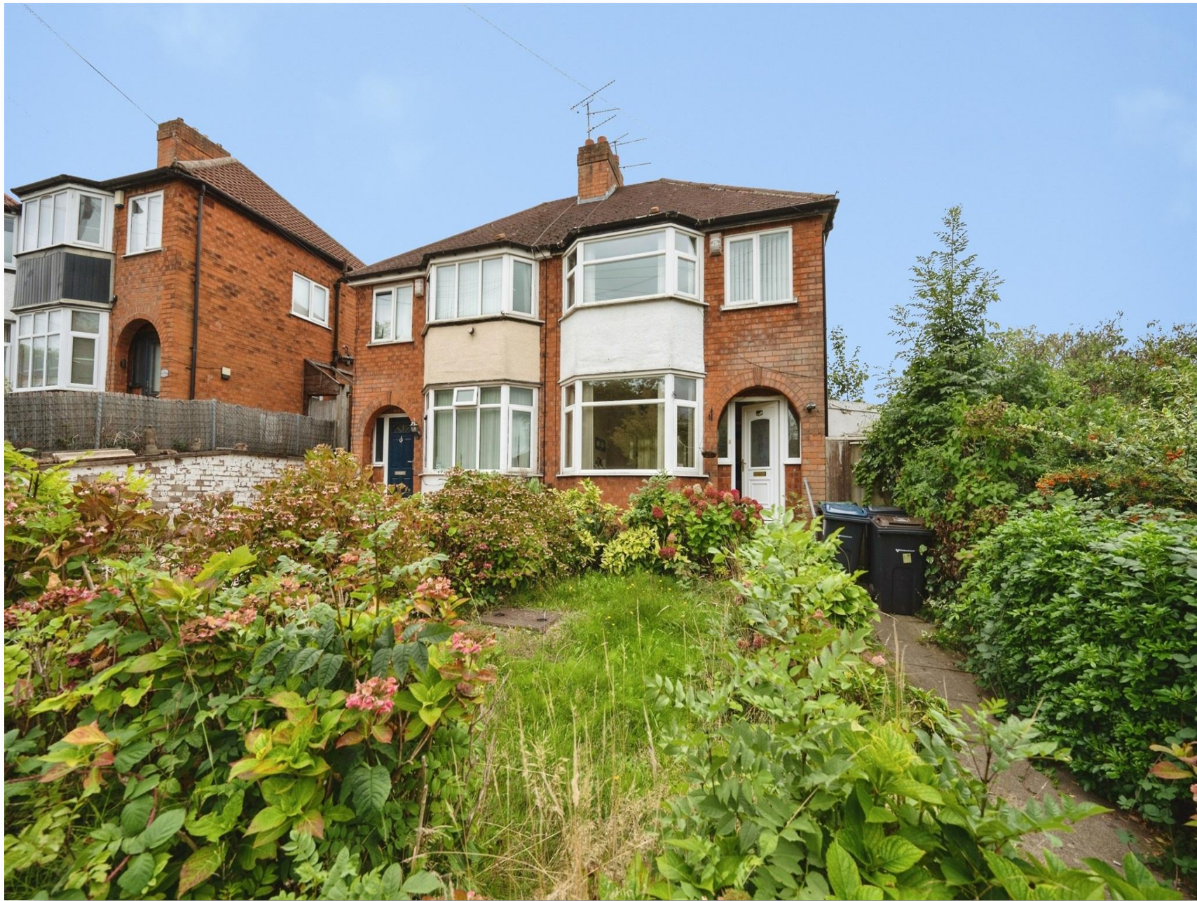
Stanford Avenue, Birmingham B42 1JT
