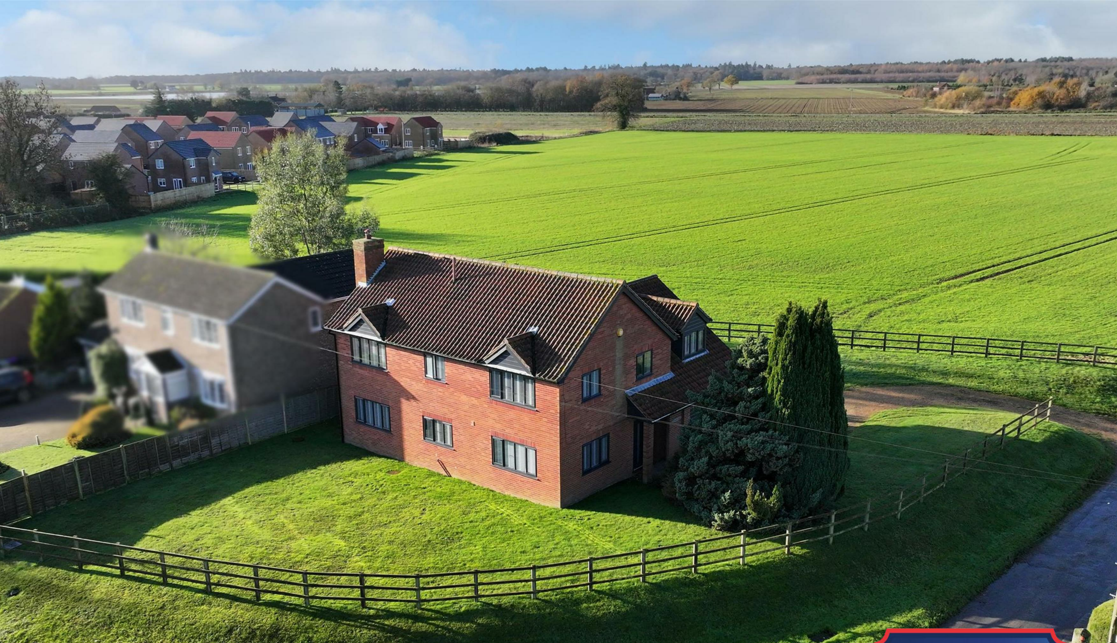
Fernleigh Manor, Watery Lane Mareham-Le-Fen, Boston, Lincolnshire, PE22 7RP
