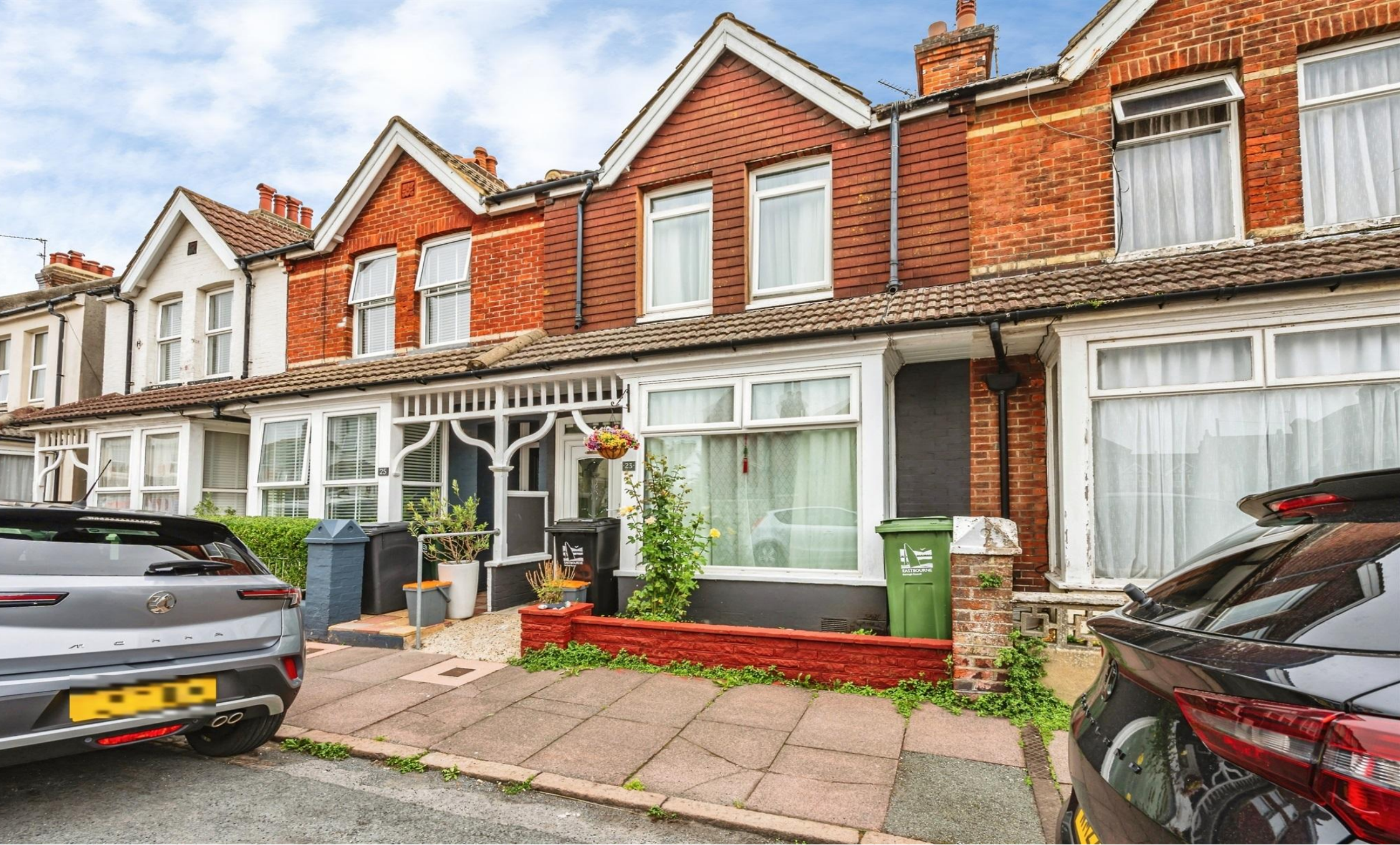
Western Road, Eastbourne BN22 8HP
