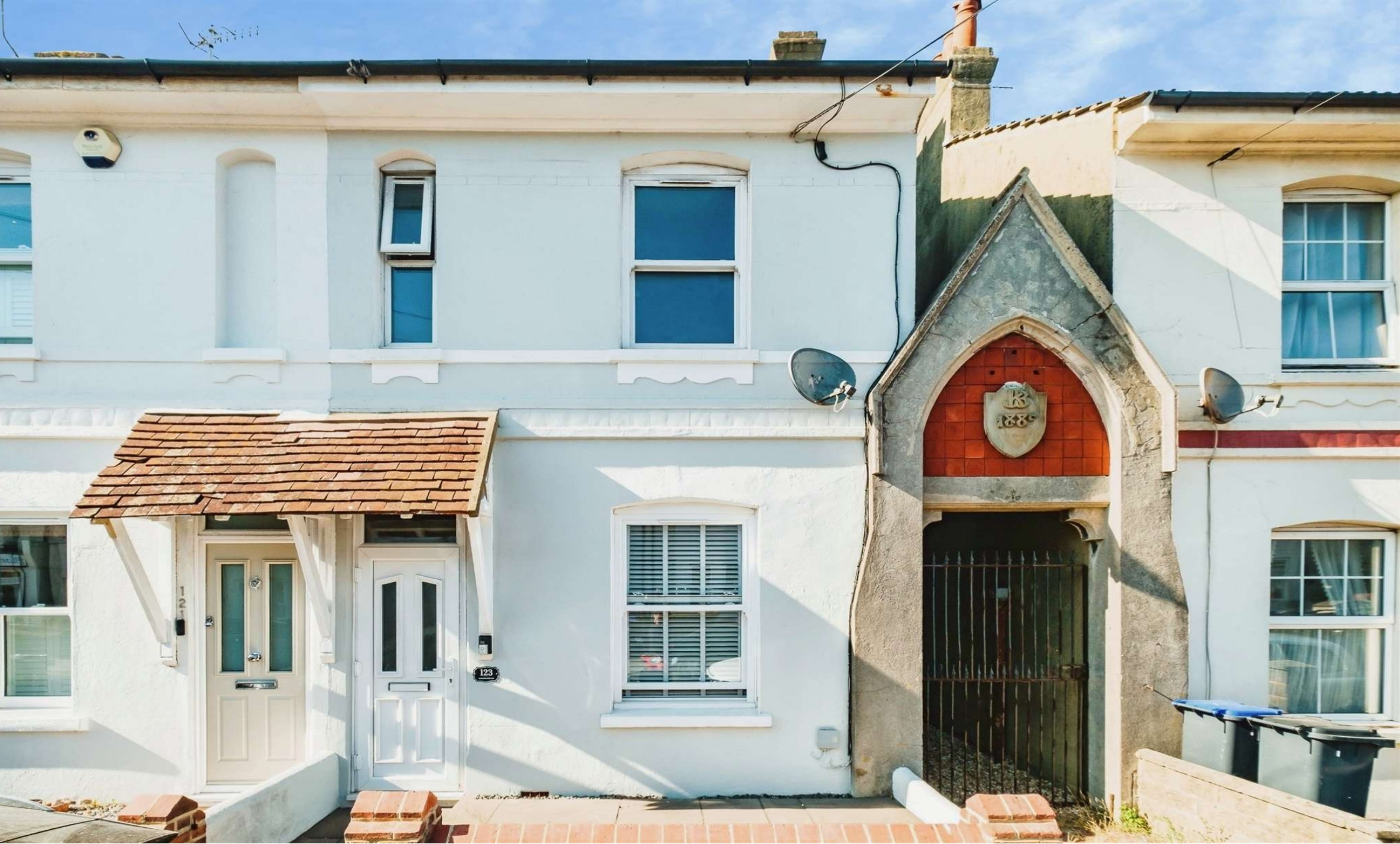
Broadwater Street East, Worthing BN14 9AP
