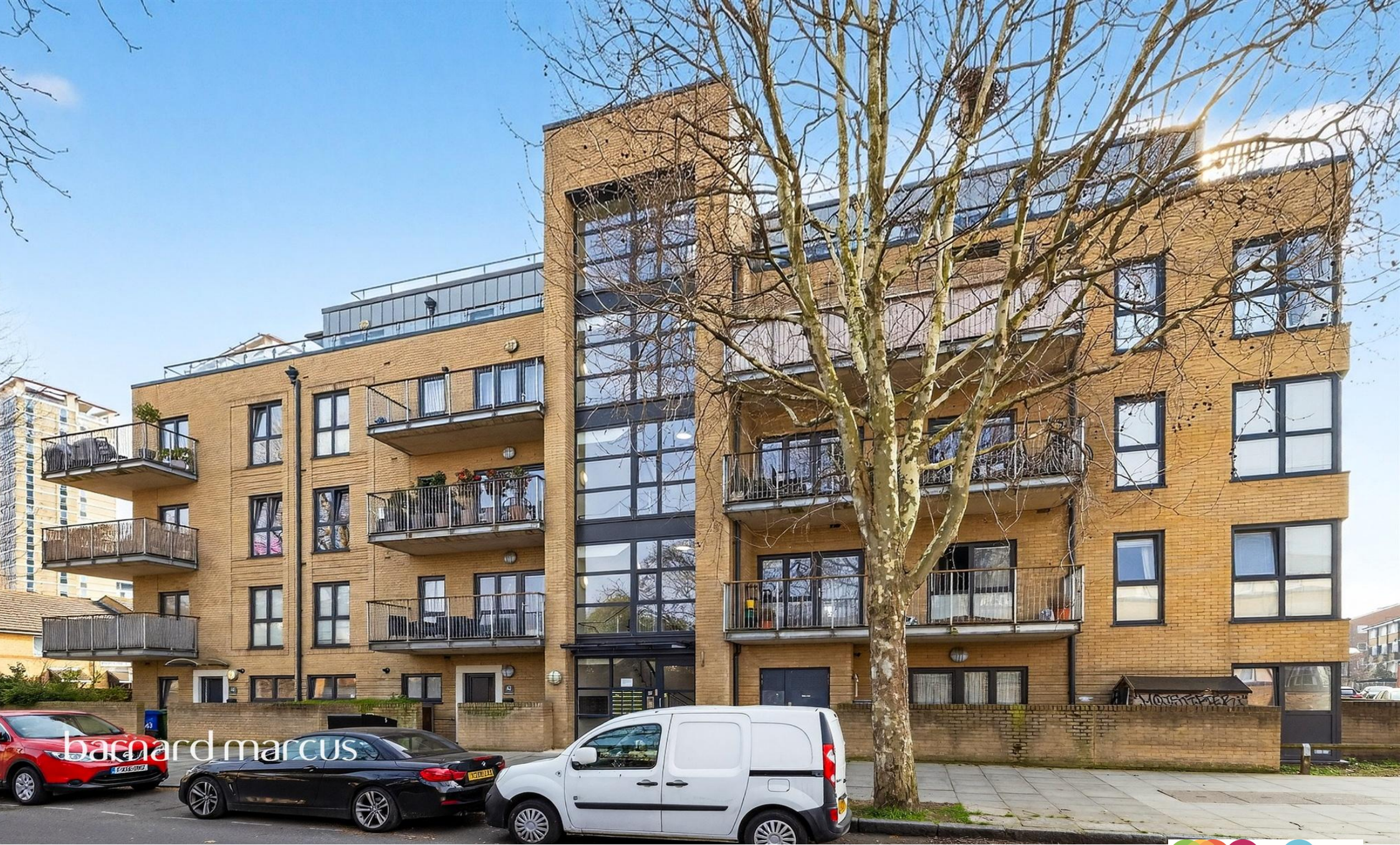
Monmouth Court Coopers Road, London SE1
