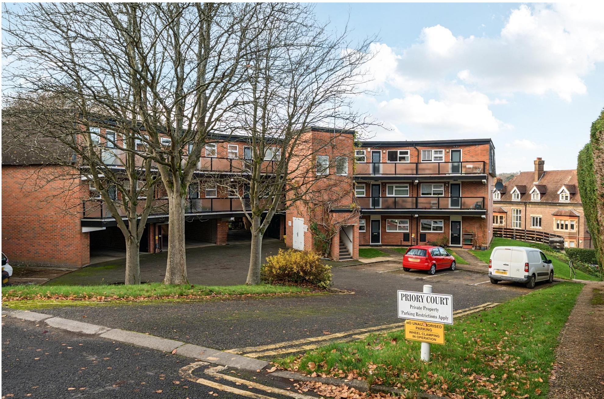
Priory Court, BERKHAMSTED HP4 2DP
