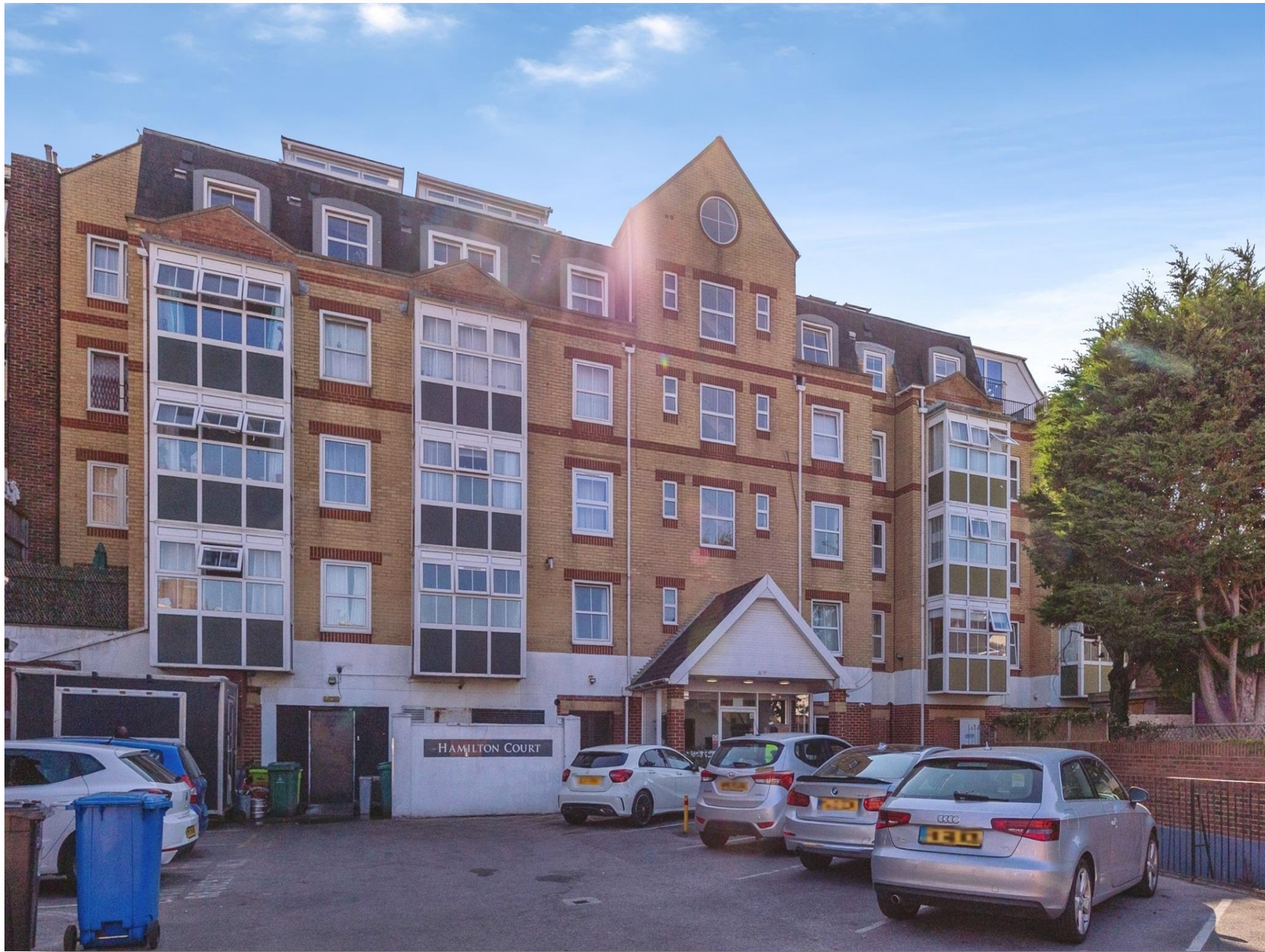
Hamilton Court Ashby Place, Southsea PO5 3NP
