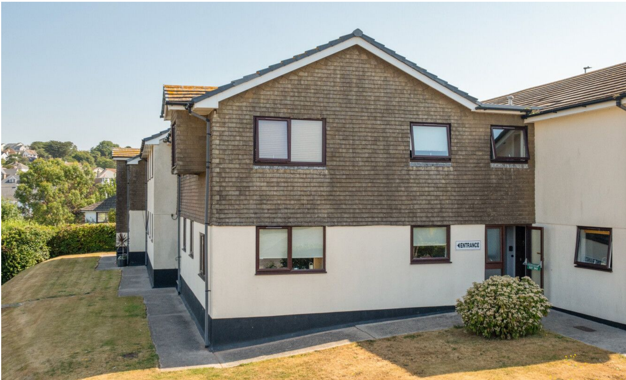
Saffron Court, Kingsbridge Kingsbridge
