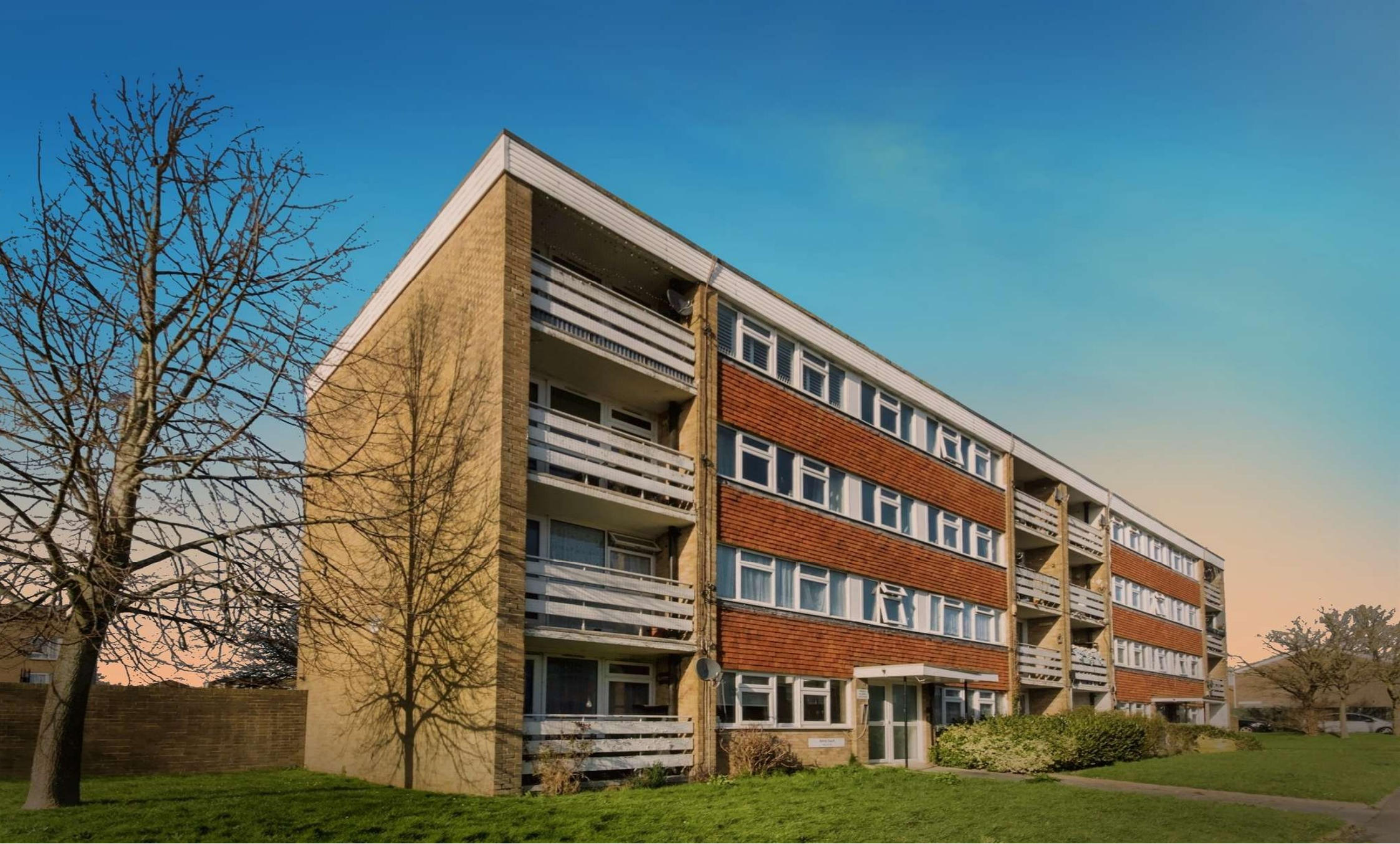
Kerry Court Westerham Road, Eastbourne BN23 7HN
