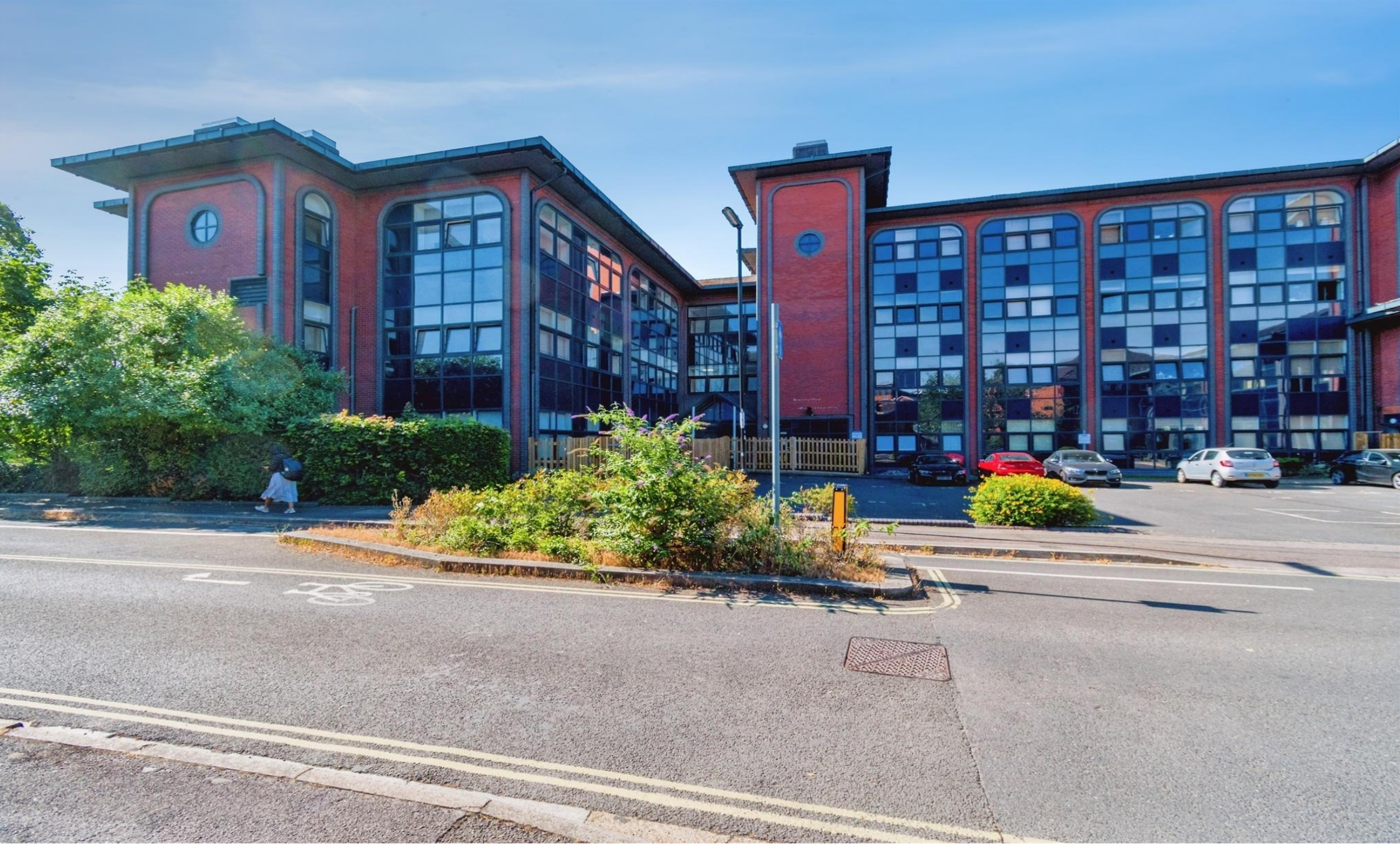
Southbrook Rise, Millbrook Road East, Southampton SO15 1BX
