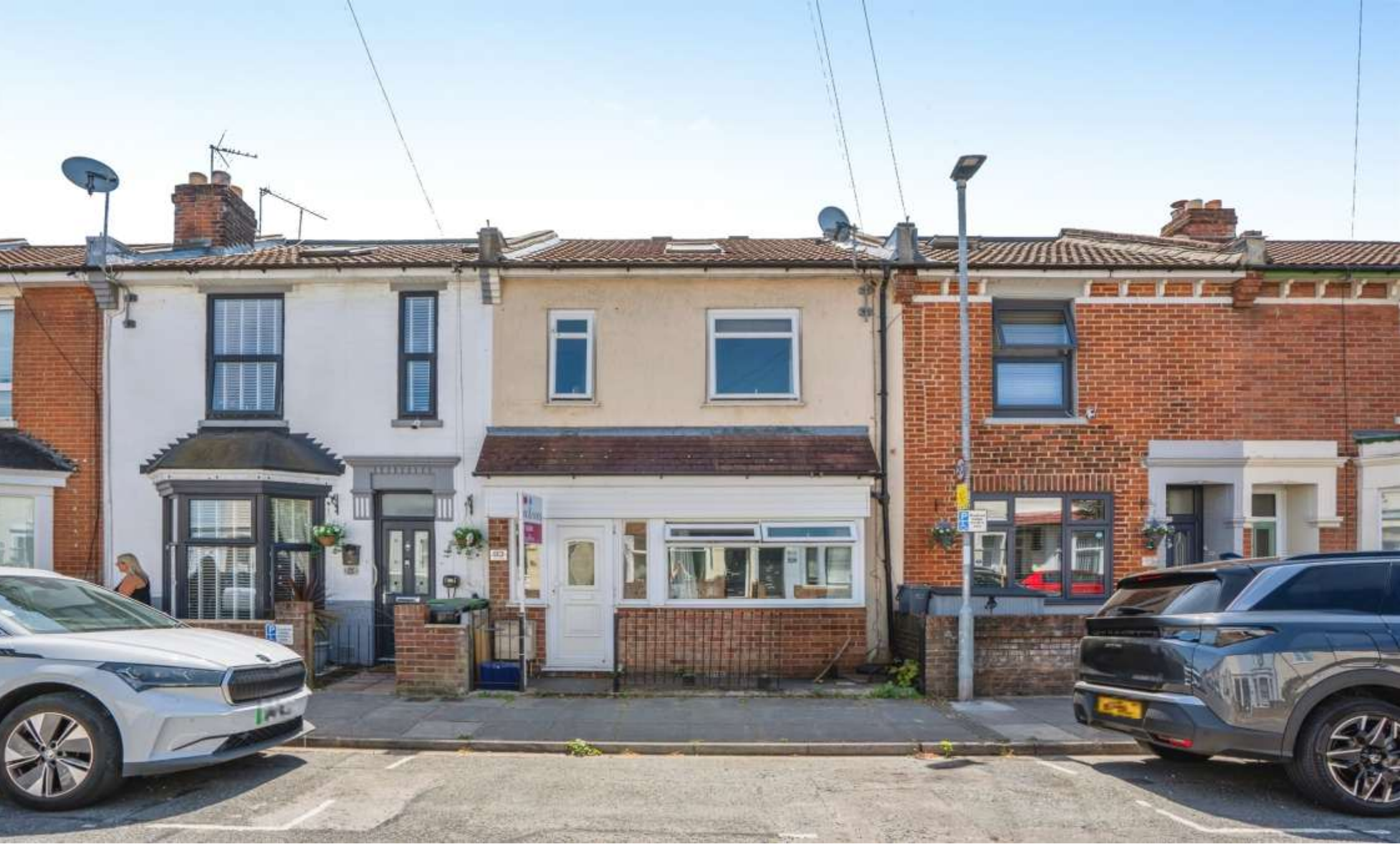
Knox Road, Portsmouth PO2 8JJ
