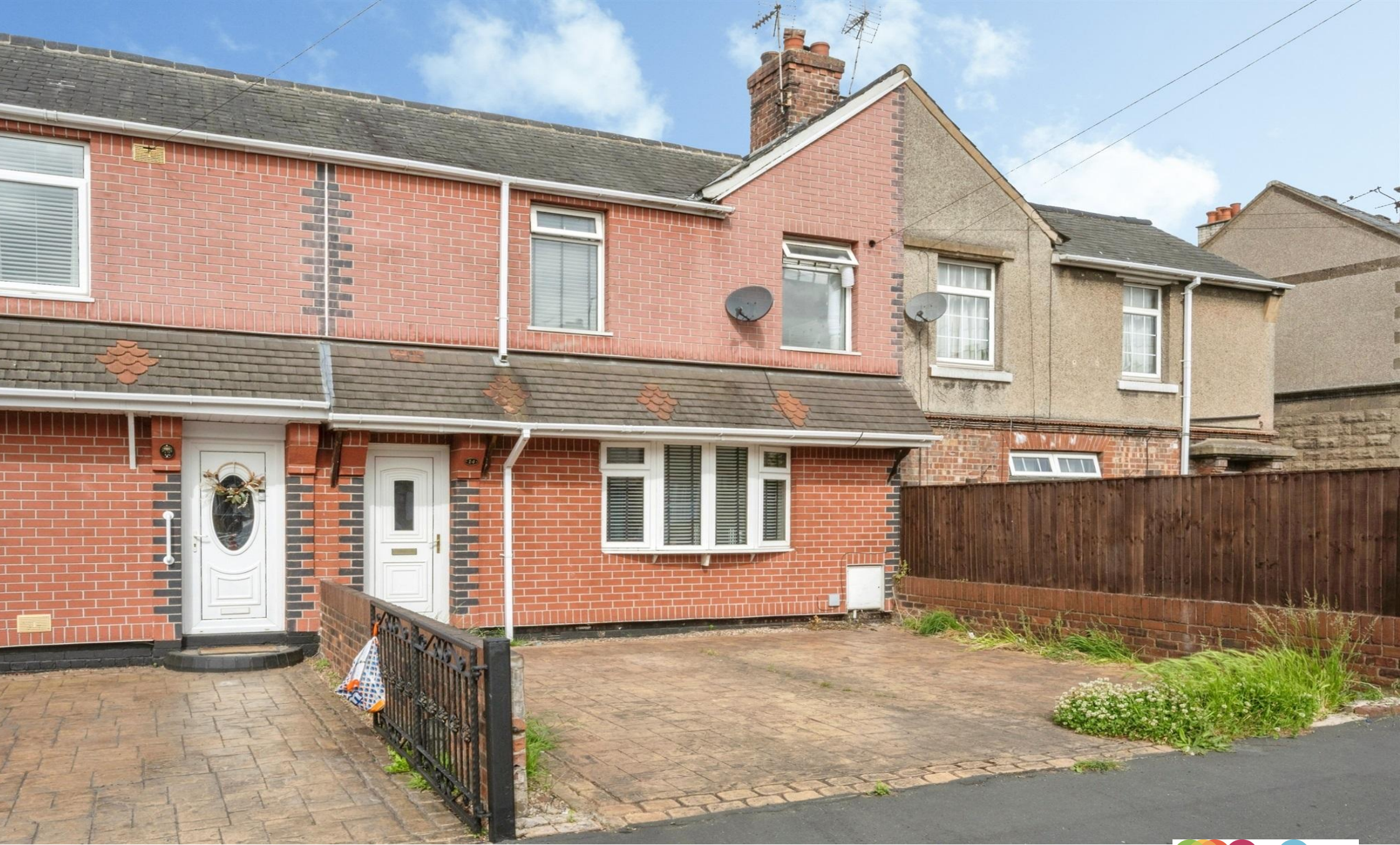
Paxton Avenue, Carcroft Doncaster
