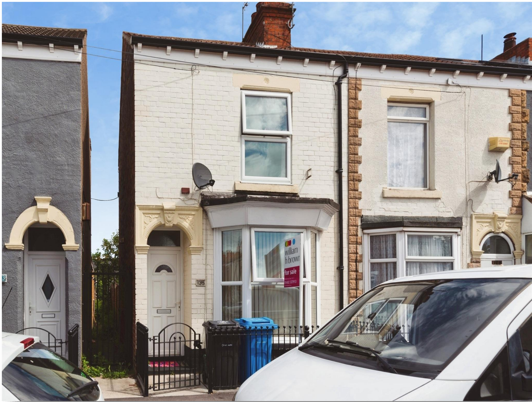
Rosmead Street, Hull, HU9 2TA
