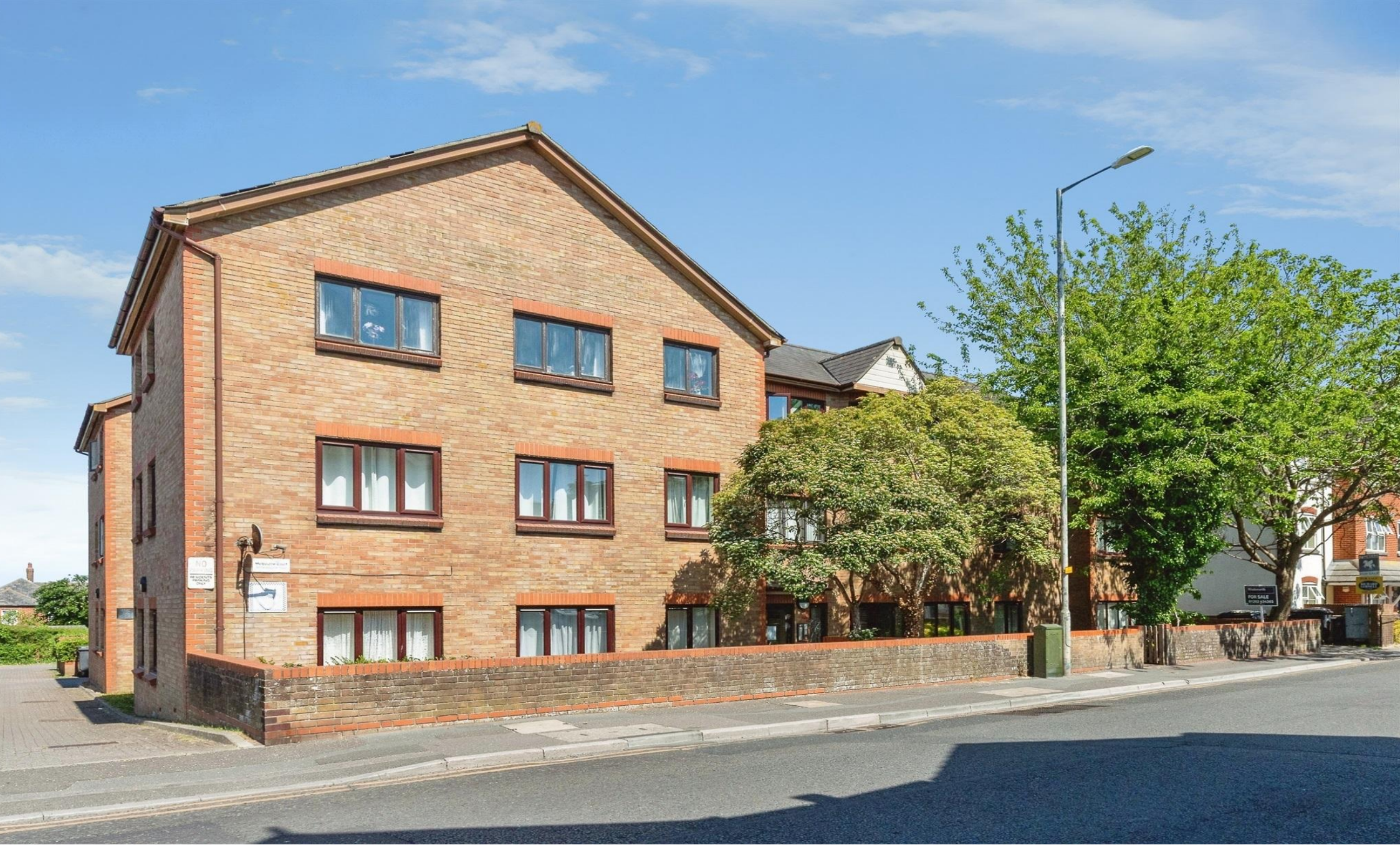
Melbourne Court Seabourne Road, BOURNEMOUTH BH5 2HT
