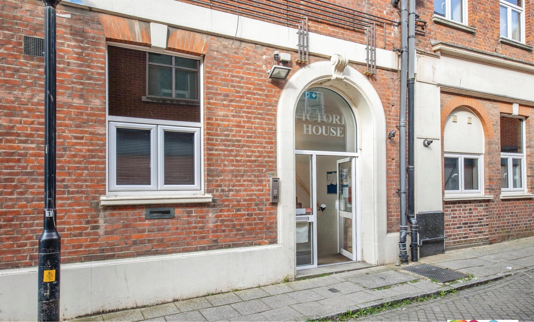
Victoria House, Eld Lane, Colchester, CO1 1PE
