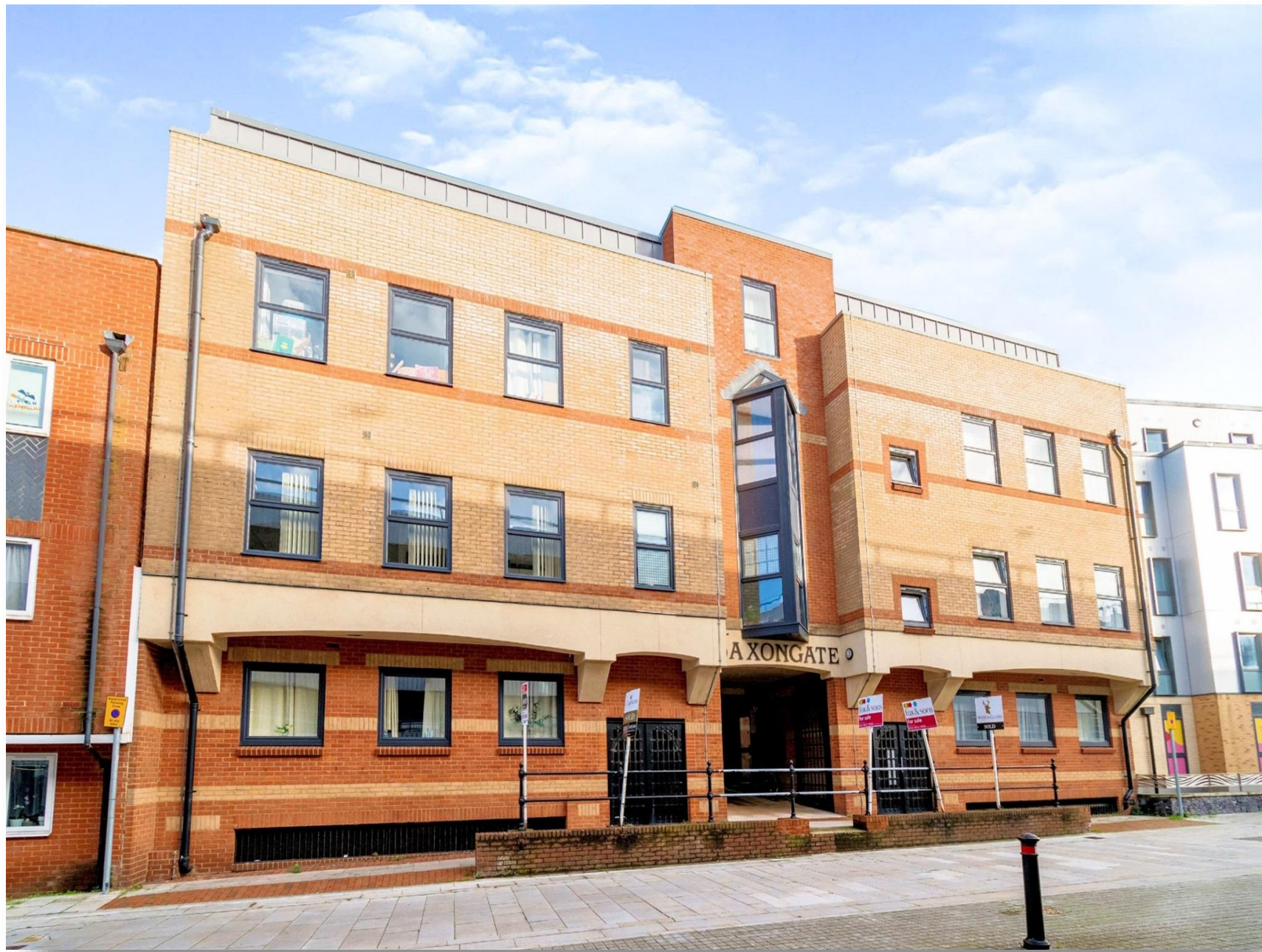
Saxon Gate, Southampton SO14 3HA
